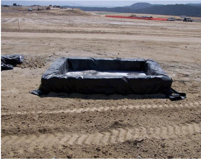
CONCRETE WASHOUT
