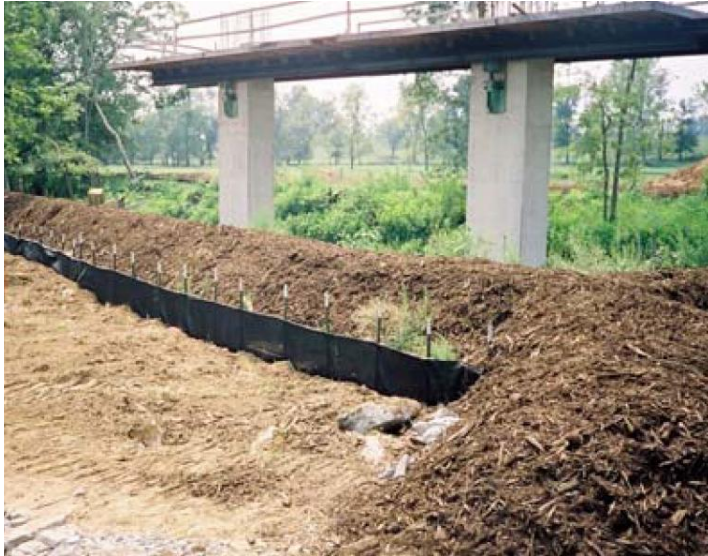
Filter berm installed with silt fence to prevent mulch migration (Source: TDOT, SR840, Williamson County)
