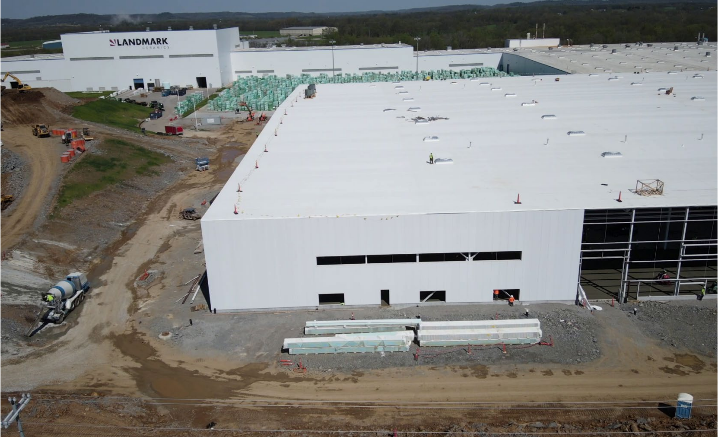
Construction continues on the expansion of Landmark Ceramics
